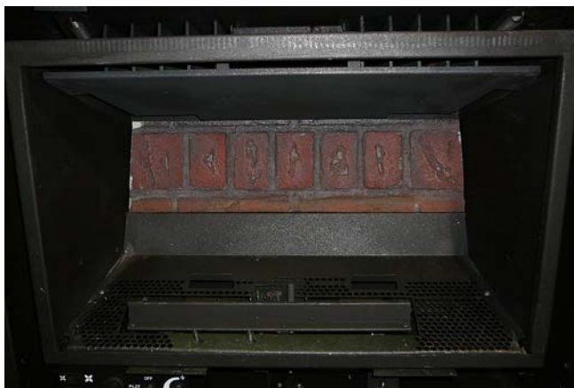
Figure 57: Back Brick Panel in Place.
