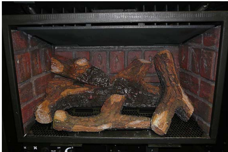
Figure 63: Fourth Stage Log Set Installation.
